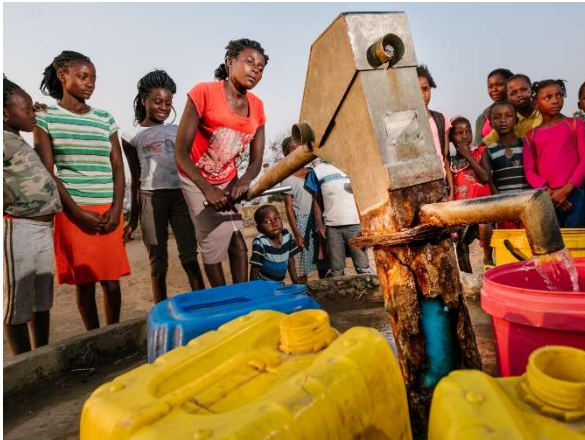
As shown on the pictures : The water has such a high level of salinity in the village that it attacks the hand pump and forces the population to use brackish water or to find water elsewhere.
