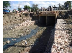
Setting of gabions along river Ng'ombe
