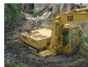
Stuck of Chain Excavator
