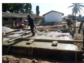
Construction of School latrines (foundation)
