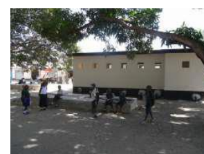
Completed School pour latrine at Mbagala Kuu
