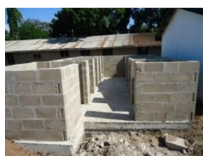
Construction of superstructure /latrine
