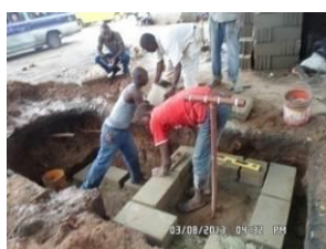
Construction of a DP
