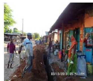
Trench digging at Kibondemaji B
