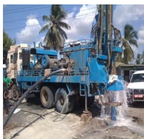
Drilling of Borehole at Mgeninani
